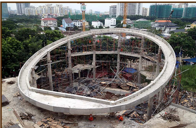
Under Construction Auditorium
