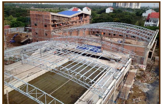
Indoor basketball court and swimming pool
